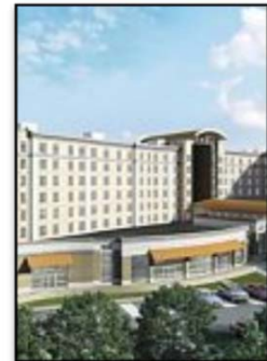
Figure 2.2: Facade. (Photo taken from Miller Global, LLC website)
